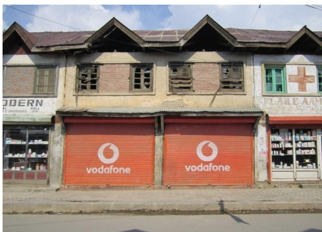
Fig. 4: Two abandoned shops of Bhoris in the main market of Bandipora town.
